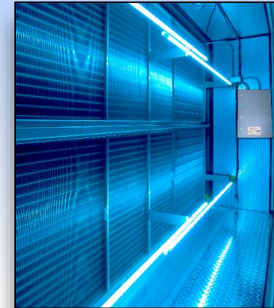
HVAC Coil/Surface Cleaning
